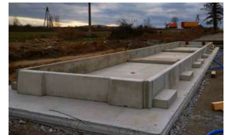
Foundations for the pit
