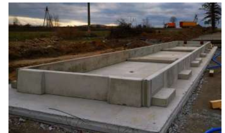
Foundations for the pit
