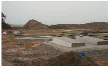
Prefabricated Foundations
