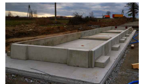
Foundations for the pit
